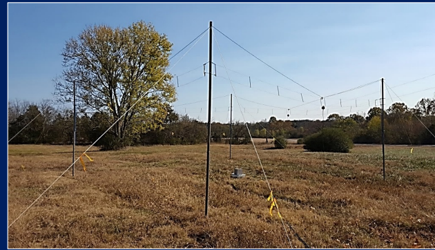
A Terminated Folded Dipole (TFD) Square Array
