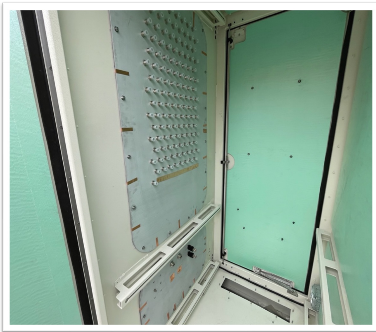
RF-IN Bulkhead connecting open compartment to ARX compartment
