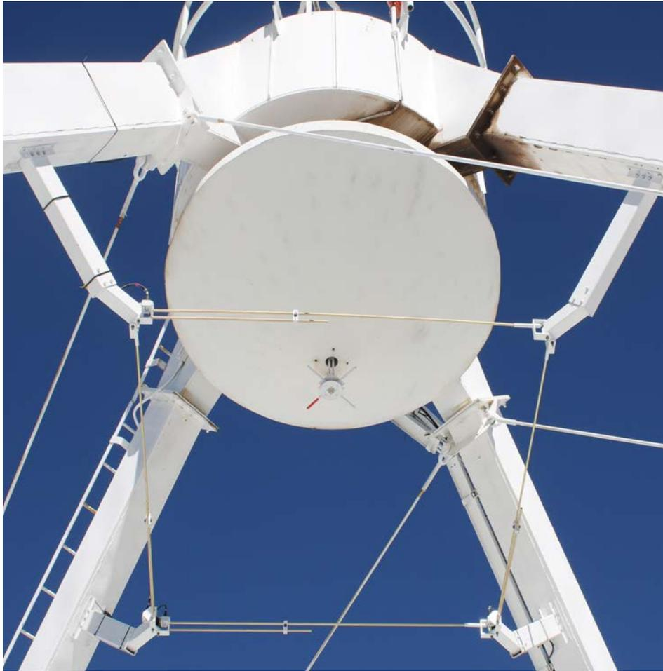
**All 28 VLA antennas equipped with MJP dipoles**
