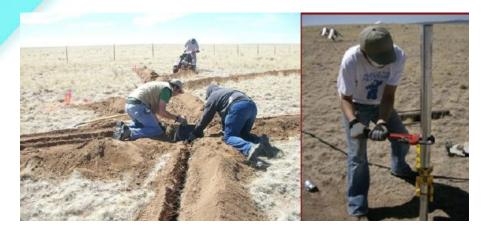
Spring Break 2009 at U. of New Mexico = Work Week at the LWA for several graduate students from the Department of Civil Engineering. They trenched, installed conduit and pulled electrical cables through it, surveyed, and tested the strength of the *Oz-Post* on which the antenna is mounted.
