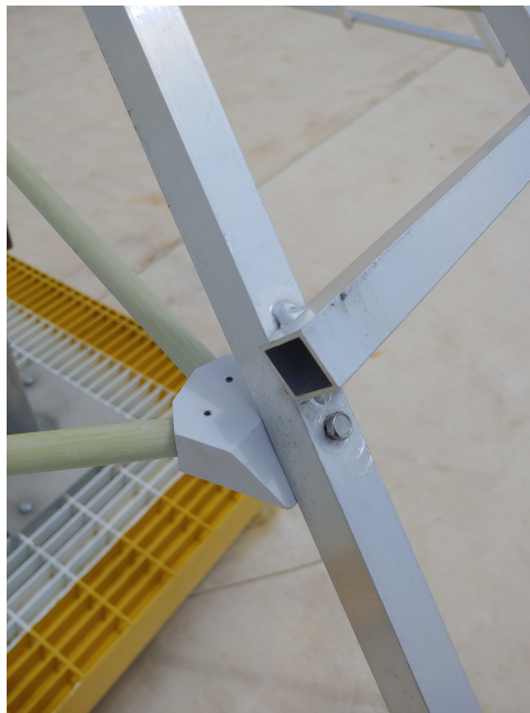
Figure 4: Junction of the antenna arm with the fiberglass support structure. The angle of the support and antenna arm should match, as seen here, and screw in without difficulty.
