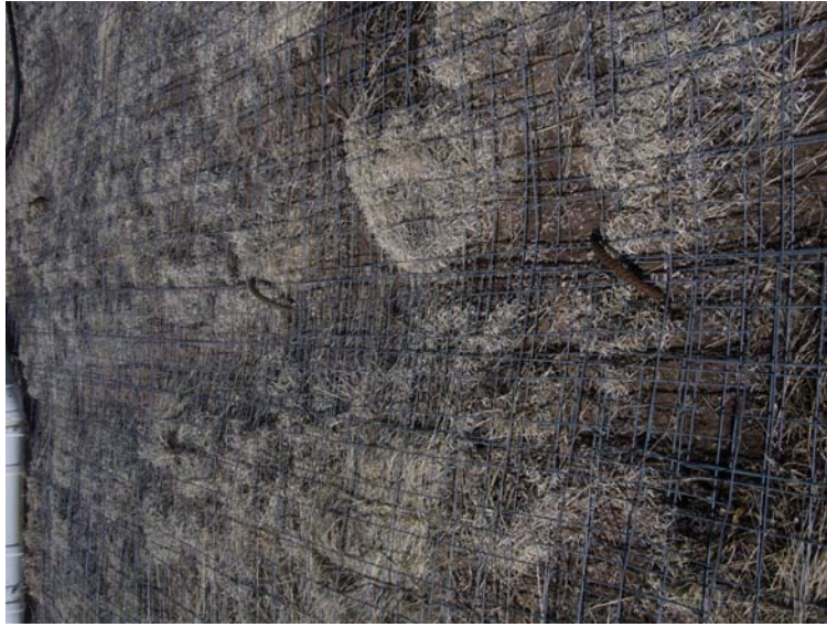
Fig. 1. Close-up of the 10mx10m ground screen. Two rebar pieces used to pin the ground screen down can be seen near the center of the image.
