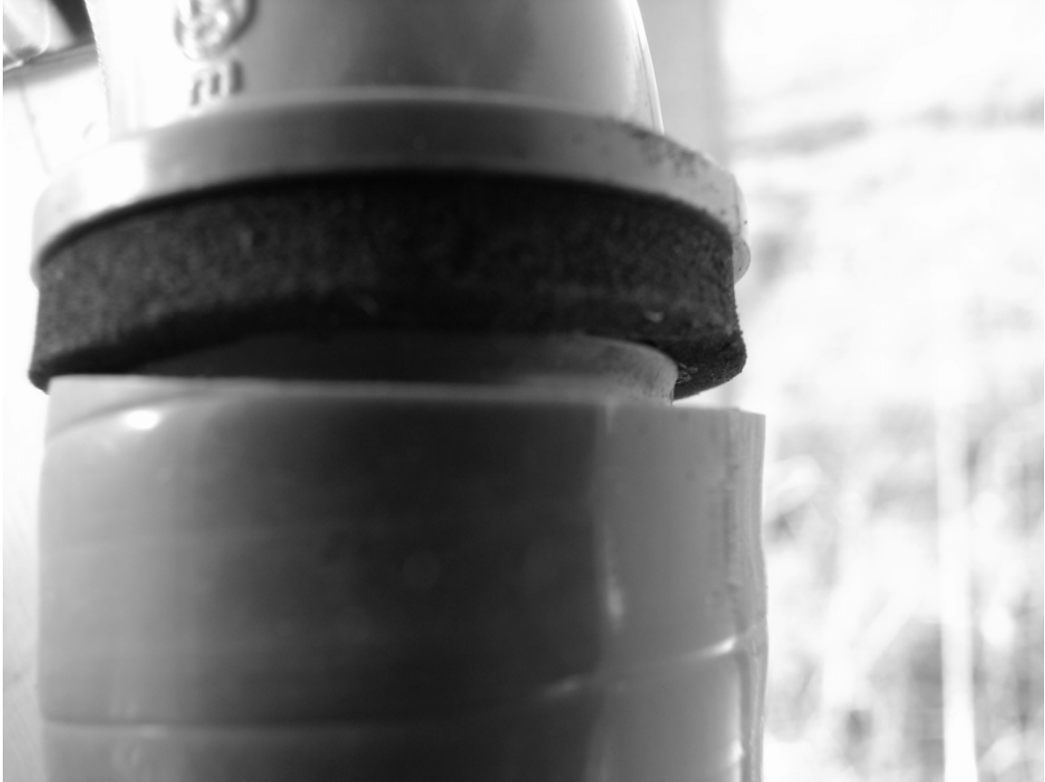
Figure 11: Example of sealant coming loose at conduit joint.
