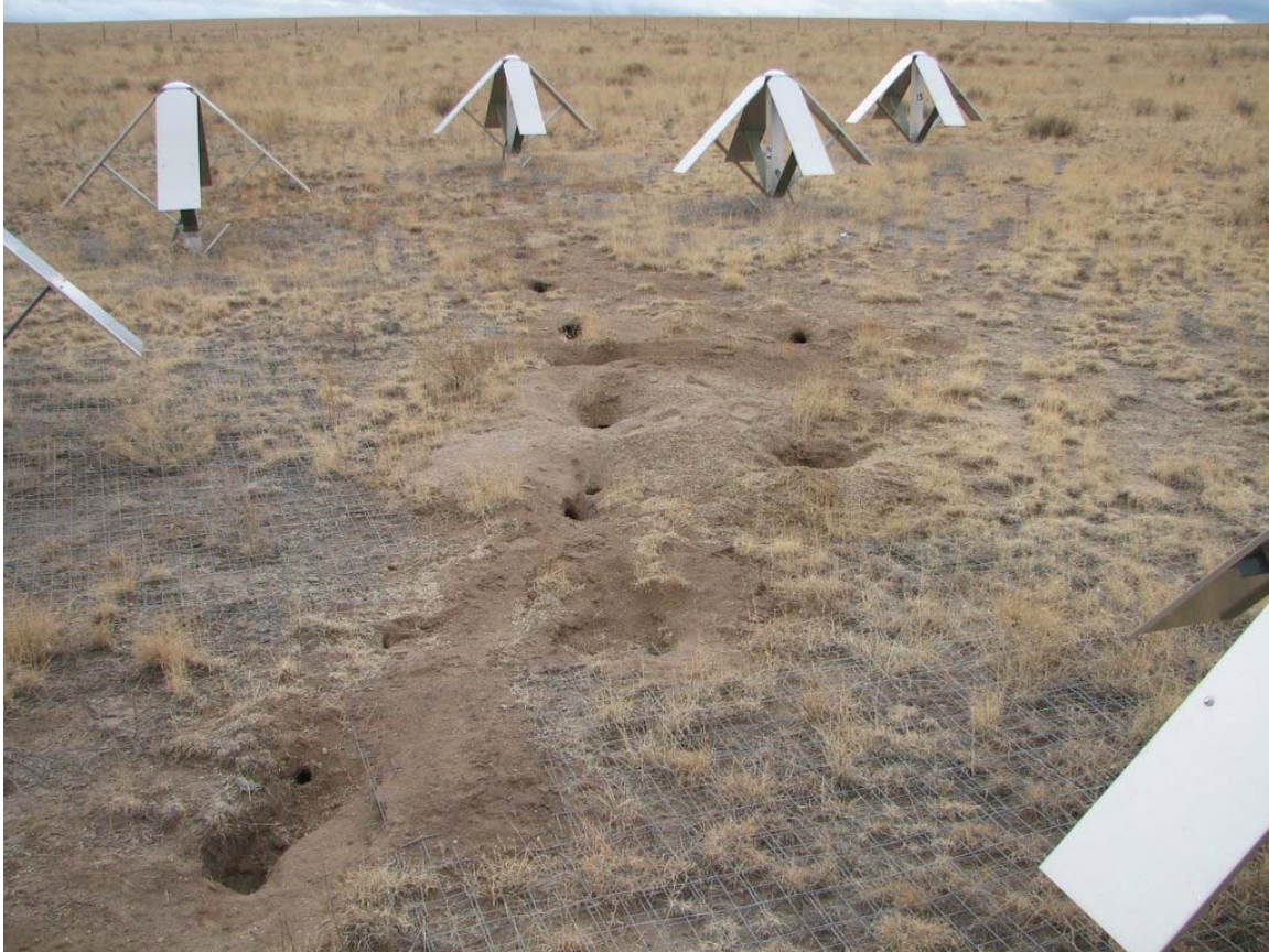
Figure 8: Example of digging activity near the center of the LWDA site. There is currently no evidence of any damage, either above or below ground, to the conduit-protected cabling associated with the LWDA.
