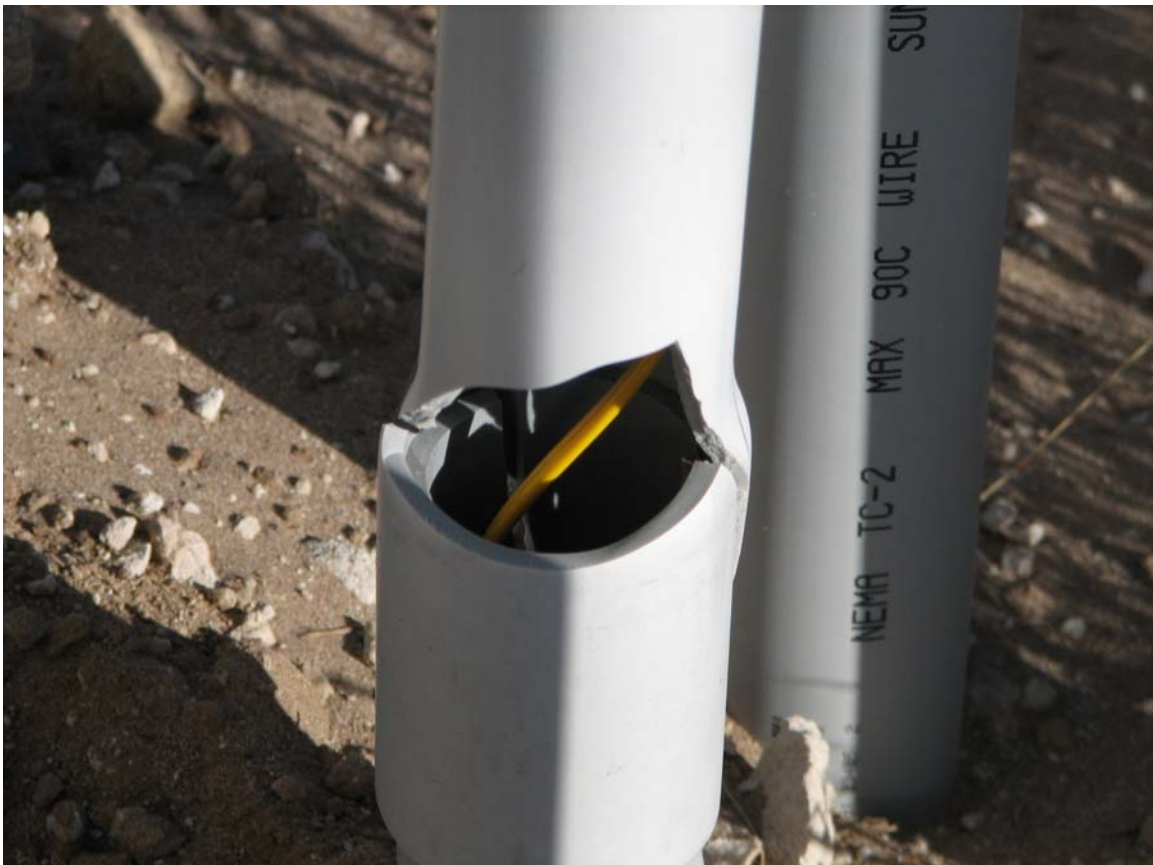
Figure 9: Broken PVC pipe covering incoming cables at LWDA site.
