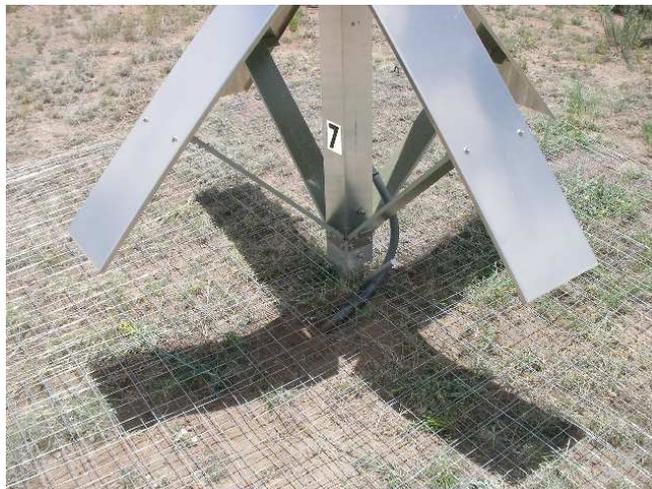
**Figure 1:** Installation of Ground Screens at the LWDA
