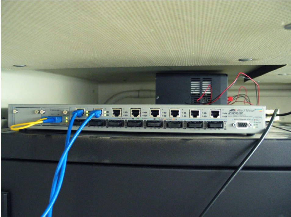
Fig. 2.— The AT-8088/SC network switch in the shelter.
