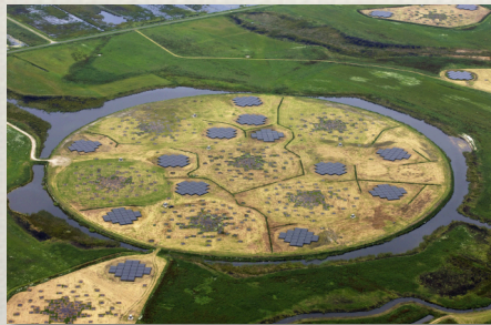
Station signals collected in the station cabinets
