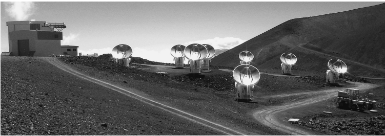
Fig. 9.9 The Sub Millimeter Array (SMA) consists of eight 6-m antennas that are designed to operate to 0.3 mm, with a total geometric collecting area is 226 \text{ m}^2 . The SMA is located on Mauna Kea, at an altitude of 4.1 km. It was built and is operated by the Harvard-Smithsonian Center for Astrophysics (CfA) and the Academia Sinica Institute for Astronomy & Astrophysics (ASIAA), Taiwan (photo courtesy of N. Patel, CfA.)
