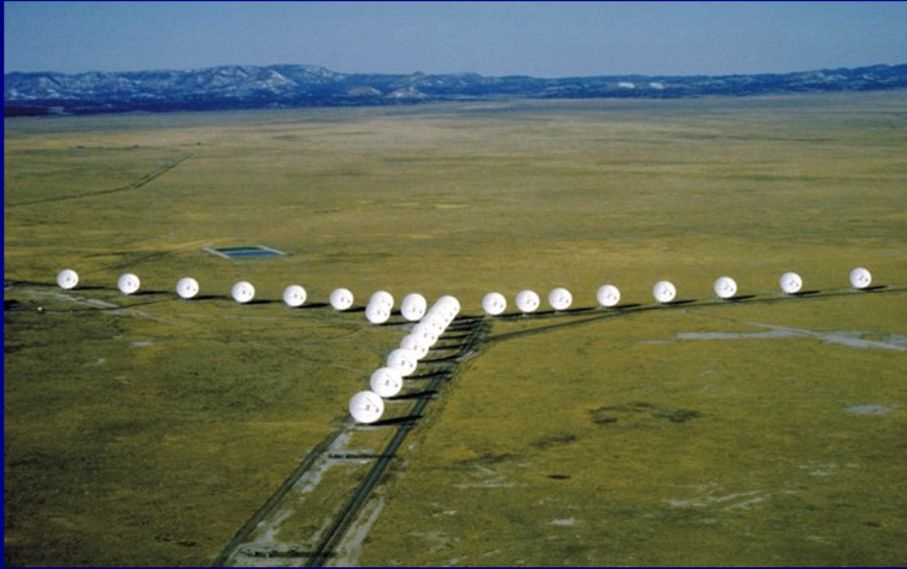
Very Large Array (NM). Maximum separation of dishes: 30 km
