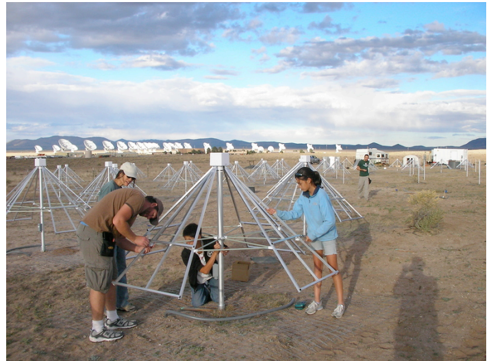
Fig. 5. Staff and students build an LWA1 antenna.
